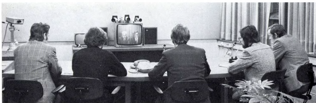
Fig. 2. Conference by video telephone. Conference stations have been installed at several points in the experimental network. In the experimental station shown here (at Philips Research Laboratories) only a single large monitor is used; the other conference stations employ several ordinary video-telephone sets.
